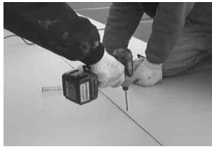
Fix by drilling screw
