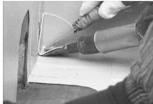
Hot blast welding (Hand-operated-Corner)
