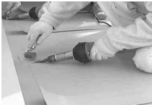
Hot blast welding (Hand-operated-Flat place)
